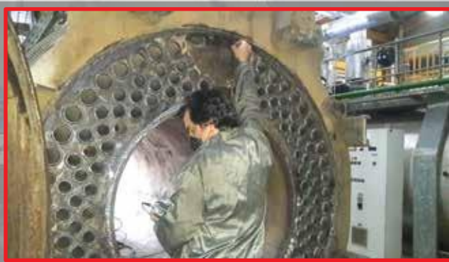
Boiler Hydrostatic test
