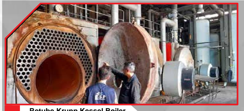
Retube Krupp Kessel Boiler
