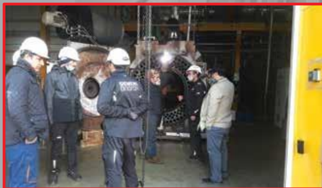
Retube Loos Boiler
