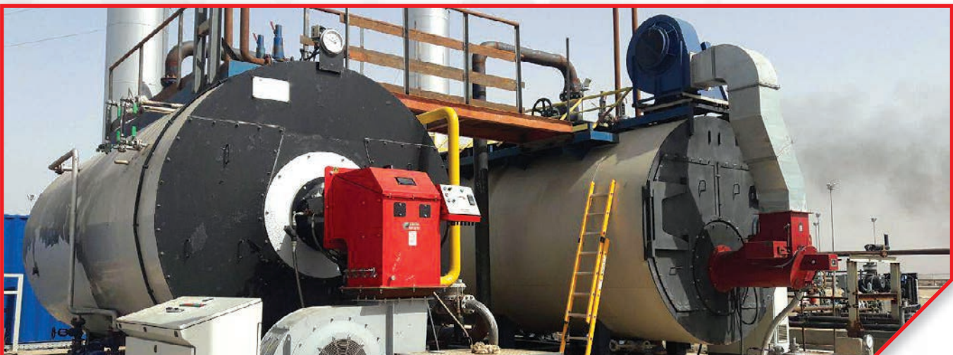
Italian Boiler and Burner Maintenance
