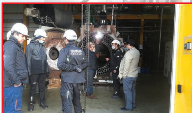
Loos Boiler Retube
