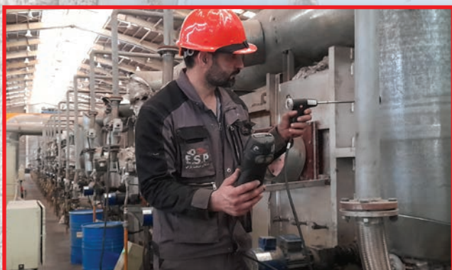
Furnace Burner Analysis
