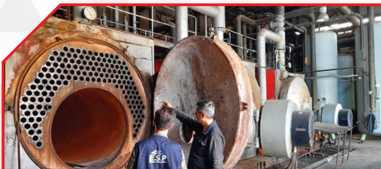
Krupp Kessel Boiler Retube
